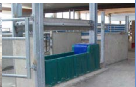
Option I: 1x MAXIFLOW float valve (connected to a feed pipe, shown with a frost protection heating cable 24 V, 20 W, 2 m), 1x heating element 24 V, 180 W
